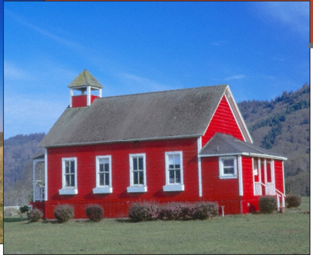
Left: The School before restoration; Above : Refurbished finished product.
